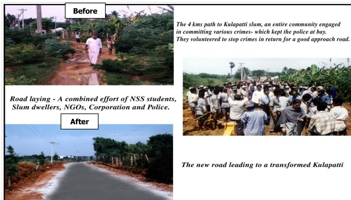
Image 8: Before and After Picture of Road Construction
