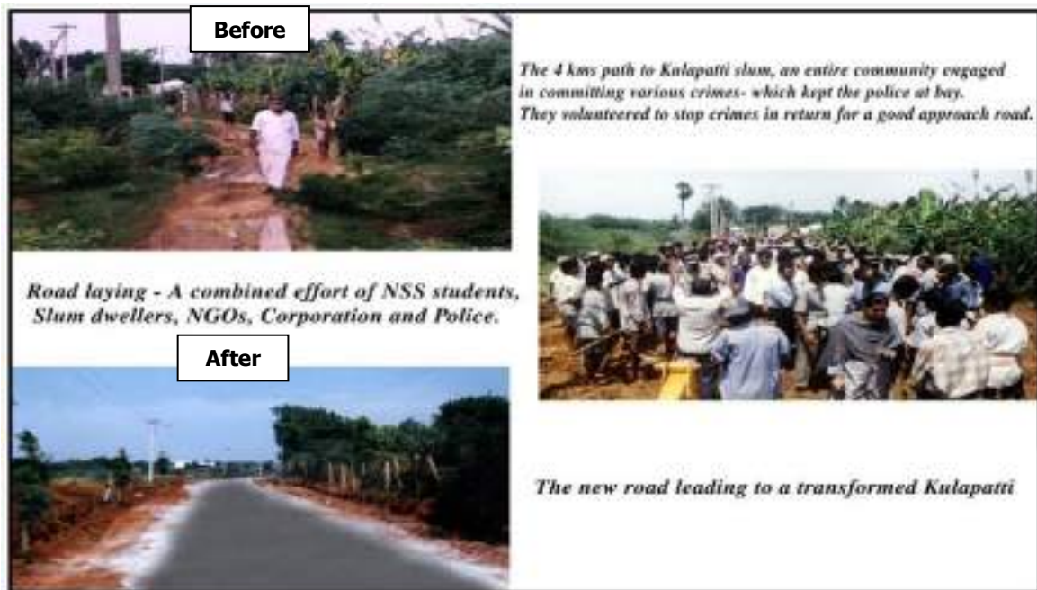
Image 8: Before and After Picture of Road Construction
